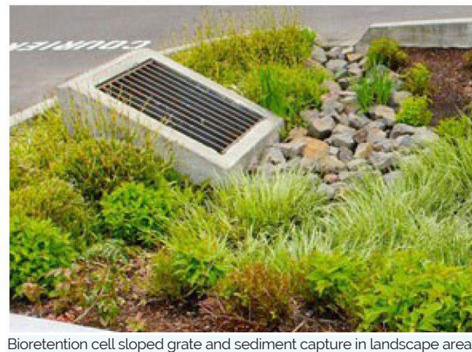
Bioretention cell sloped grate and sediment capture in landscape area.
